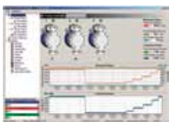
Fig. 3: Pump status or status of each individual pump head "Traffic Light"
